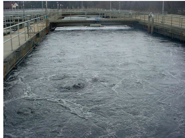
Figure 7.35 Diffused aeration system in operation.
