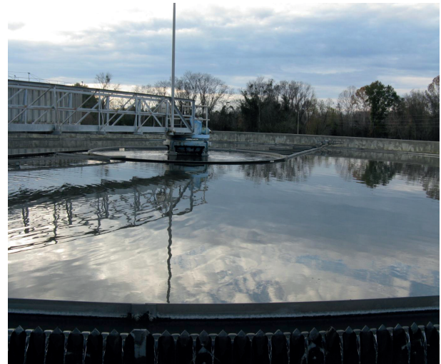
Figure 7.8 A circular primary clarifier.
