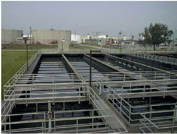
Figure 7.7 Rectangular primary clarifiers.
