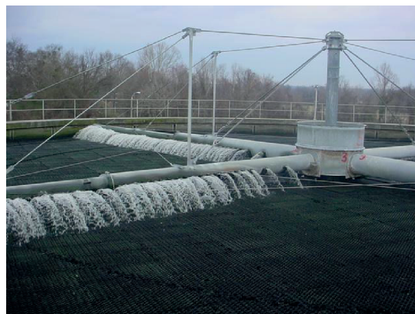
Figure 7.39 Photograph of trickling filter with plastic media.
