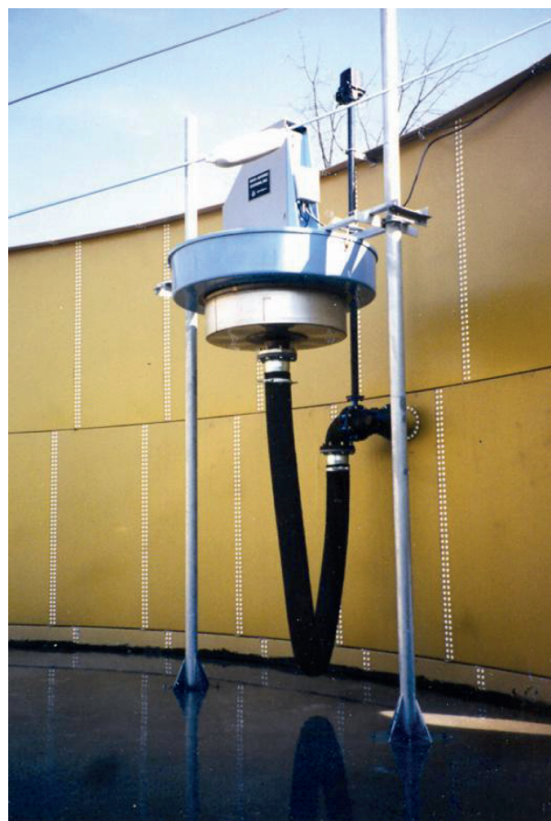
Figure 7.31 Aqua-Aerobics Decanter (hose design). Source: Courtesy of Aqua-Aerobic Systems, Inc.
