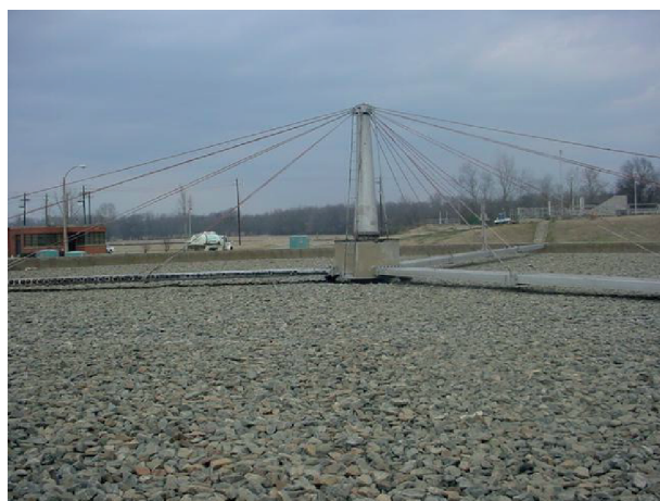
Figure 7.38 Photograph of conventional trickling filter with rock media.
