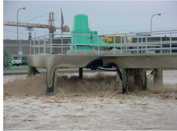
Figure 7.34 Mechanical aerator in operation.
