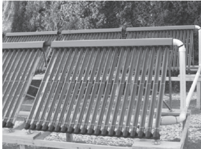
Figure 10.7 Evacuated tube collector. Source: http://www.sunmaxxsolar.com/how-evacuated-tube-solar-collectors-work.php . © Hickory Ridge Solar.
